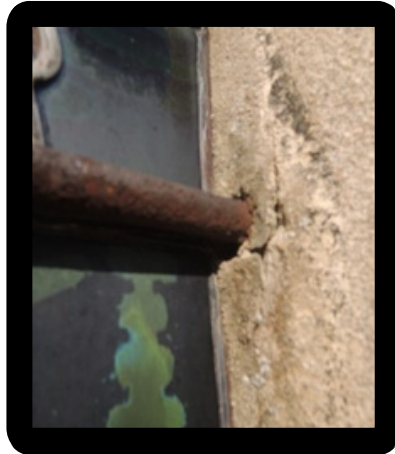
Spalling of stonework (rusting iron works)
