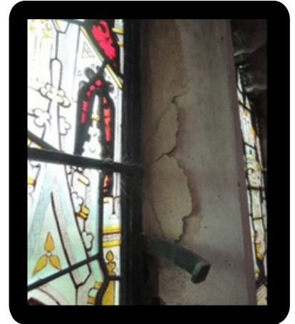
Crumbling stone work (rusting metal bars)
